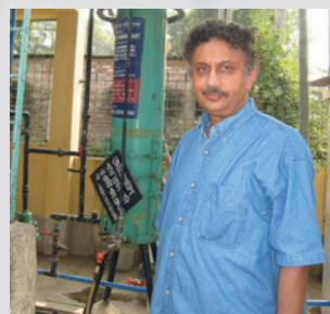
Arup SenGupta's first Sustainable Arsenic Removal System was installed in India in 2004.
