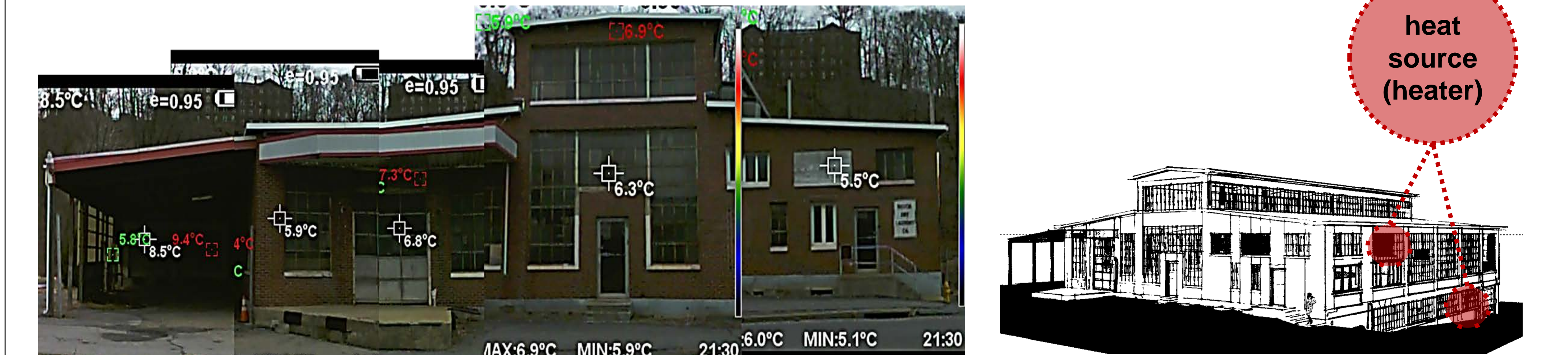
Figure 4: South Façade Photographs – Compilation
