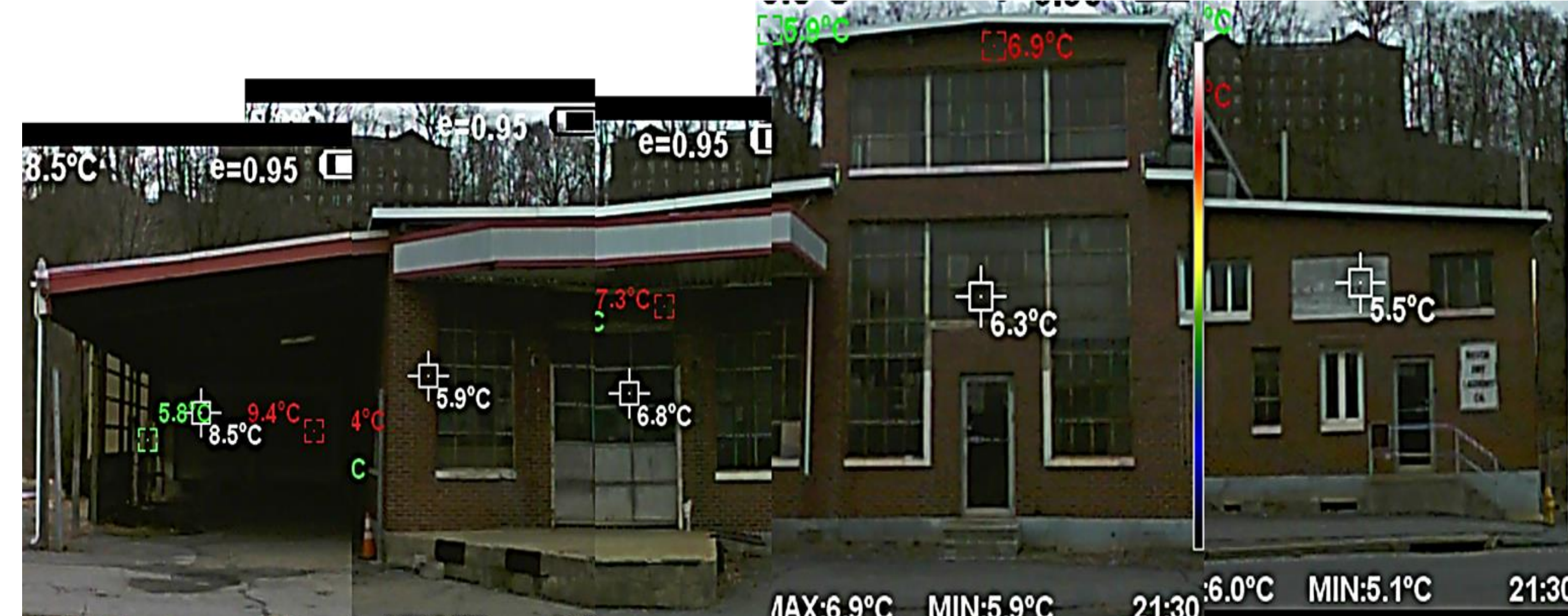
Figure 4: South Façade Photographs – Compilation
